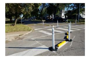
**35th and Askew:** During a traffic calming demonstration, a temporary bump out was placed near the intersection of 35th Street and Askew. The bump out, which was laid out with a set of yellow 4x4s and some plants, decreased the overall width of the roadway and indicated that drivers in the intersection need to slow down.
