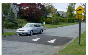
**Speed Humps** are parabolic vertical traffic calming devices intended to slow traffic speed on low volume, low speed roads. Speed humps are 3-4 inches high and 12-14 feet wide, with a ramp length of 3-6 feet, depending on target speed. They reduce speeds to 15-20 miles per hour and are often referred to as "bumps" on signage and by the general public.
