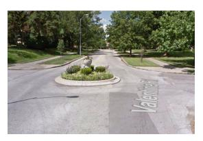
**Traffic Circle:** Also known as "mini roundabouts," traffic circles lower speeds at minor intersection crossings and are an ideal treatment for uncontrolled intersections. They may be installed using simple markings or raised islands, but are best applied in conjunction with plantings that beautify the street and the surrounding neighborhood. Careful attention should be paid to the available lane width and turning radius used with traffic circles.
